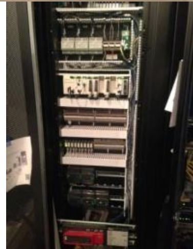
Site microgrid controller + DSO hardware
