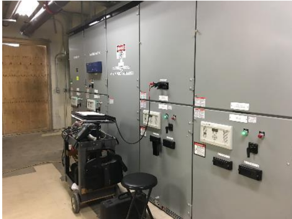
New 13.8KV Main-Tie-Main incoming utility gear
