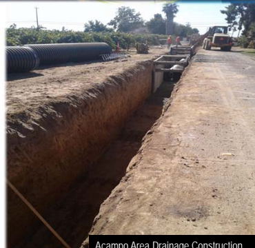
Acampo Area Drainage Construction
