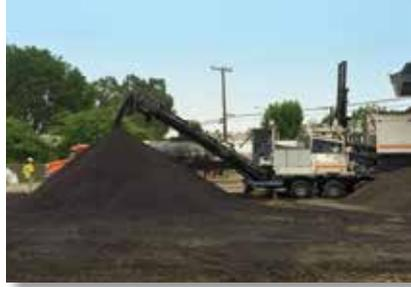
Significant benefits were achieved by using a treatment that re-uses the existing pavement and subgrade materials in place, rather than the traditional reconstruction methodology of removing the existing materials and replacing them with new pavement materials. Compared to the traditional method, the sustainable treatment resulted in:
