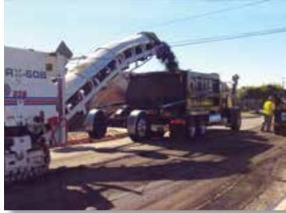
The project plan focused on reutilizing the existing materials in-place to reconstruct approximately 6 miles of residential roadways (983,000 square feet). The scope of work included paving 1.5 inches of Asphalt Rubber Hot Mix on 3 inches of Cold Central Plant Recycled Asphalt Concrete Pavement over 8 to 10 inches of Cement Stabilized Pulverized Base.
