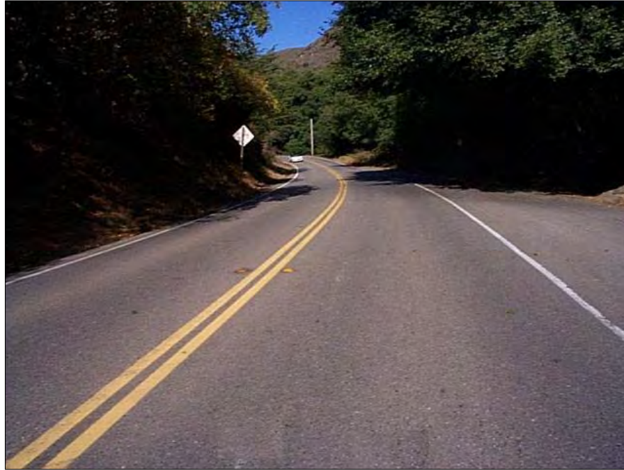
Figure 3.3 PCI = 98 (Excellent Condition)
