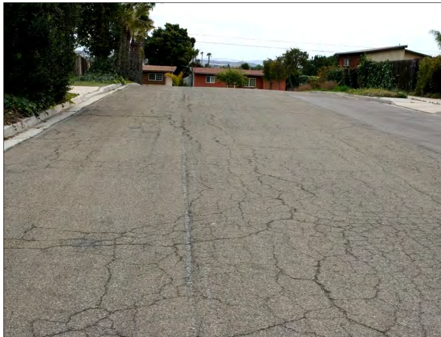
Figure 3.6 PCI = 40 (Poor Condition)
