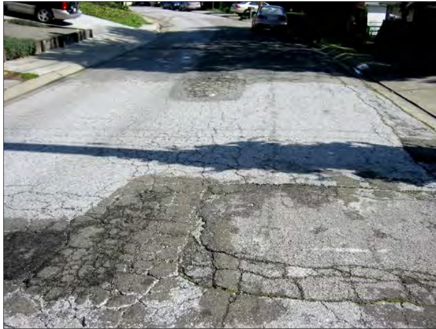
Figure 3.7 PCI <10 (Failed Condition)
