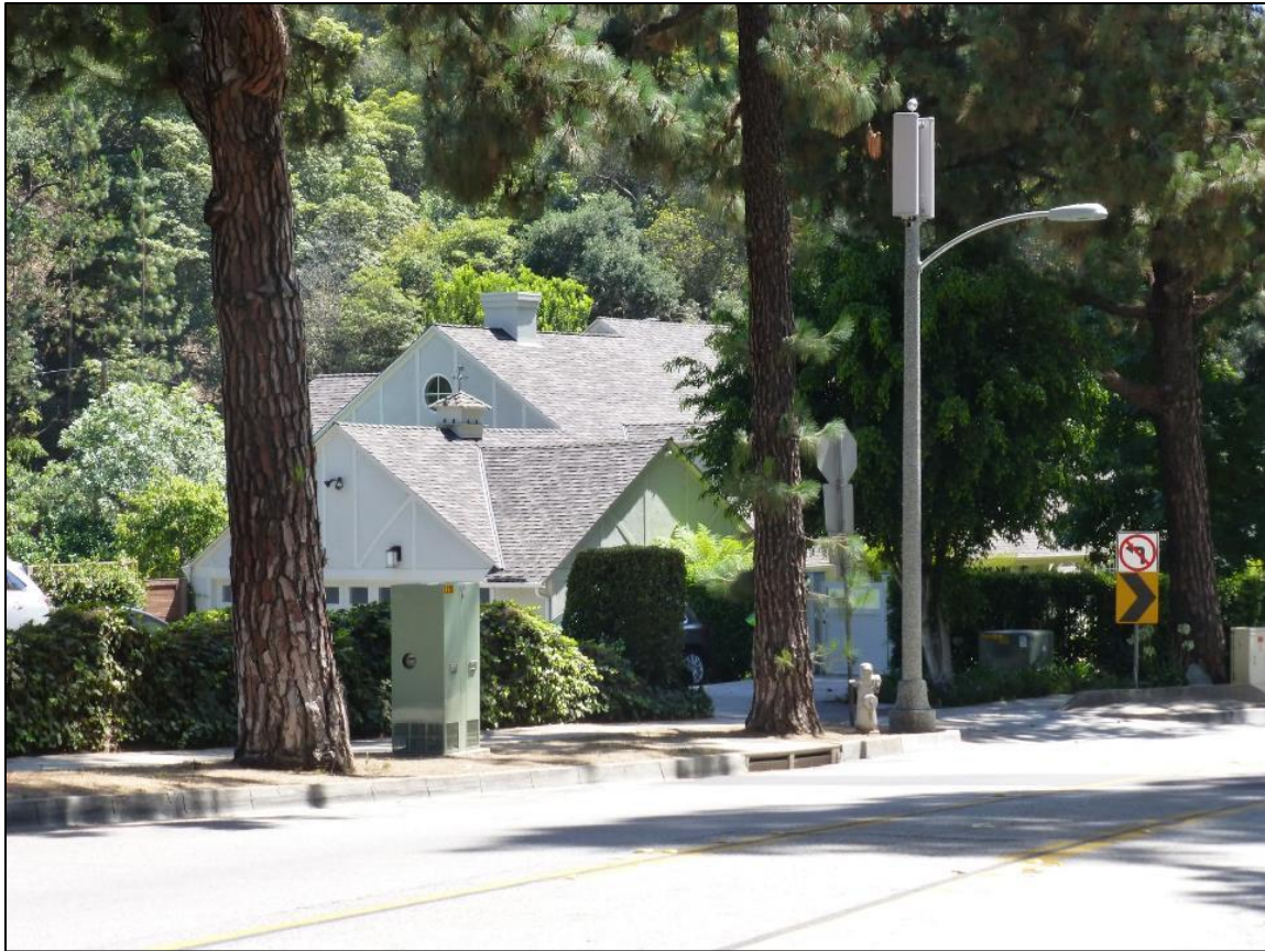
Figure 1: Sample small wireless facility on existing street light. (Photo by Dr. Jonathan L. Kramer.)
