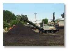
Significant benefits were achieved by using a treatment that re-uses the existing pavement and subgrade materials in place, rather than the traditional reconstruction methodology of removing the existing materials and replacing them with new pavement materials. Compared to the traditional method, the sustainable treatment resulted in:
